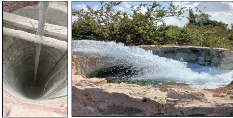
Figure 7 – Groundwater production well for irrigation in Sharqia (photos by Samar Gomaa).
